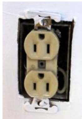
Outlets, junction boxes and fittings must have cover, faceplate or fixture canopy
