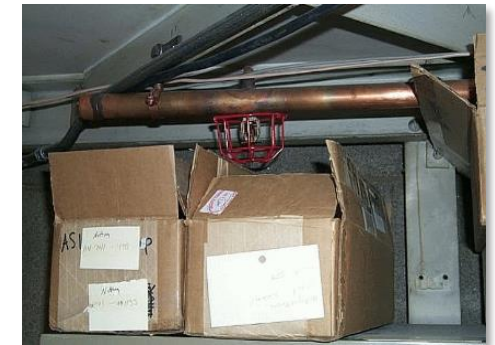
Blocked sprinkler heads
