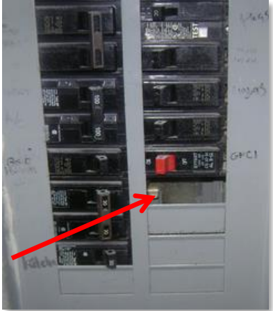
Inserts missing inside panel box
