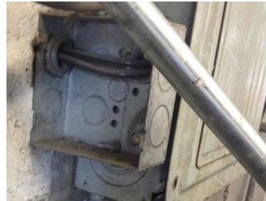
Outlets, junction boxes and fittings must have cover, faceplate or fixture canopy
