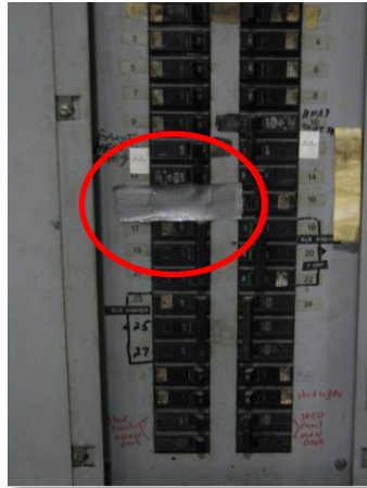
Inserts missing inside panel box
