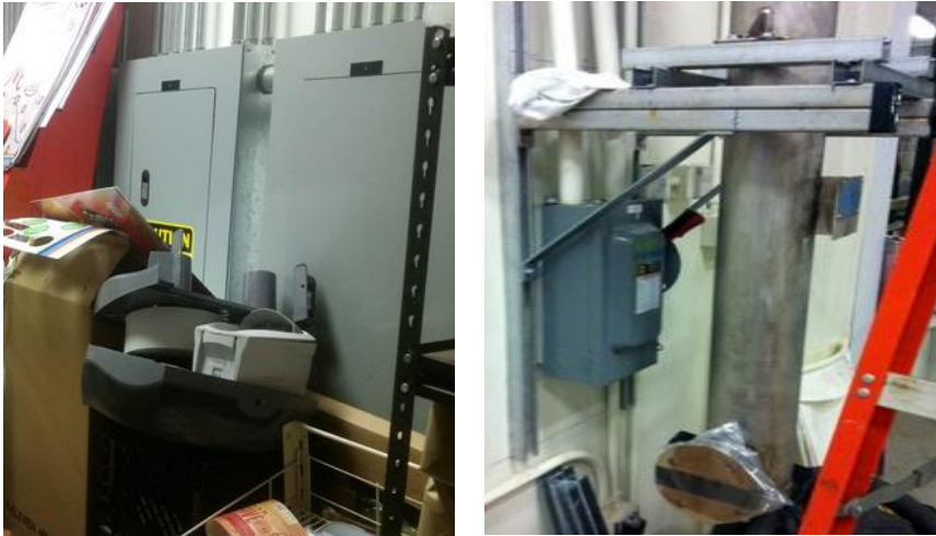
Blocked panels/switches
