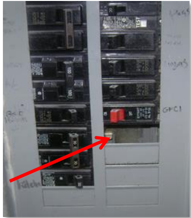
Inserts missing inside panel box
