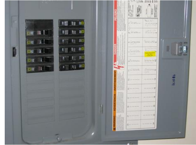
Panel and switch labeling
