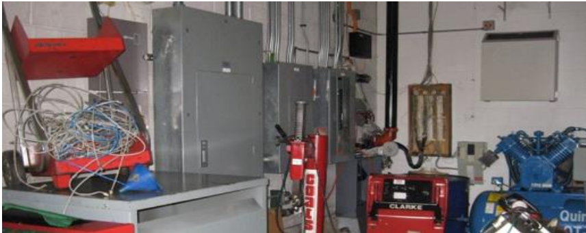
Blocked panels/switches
