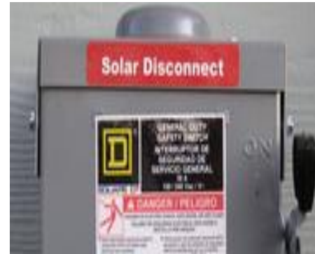
Panel and switch labeling
