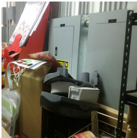
Blocked electrical panels and switches
